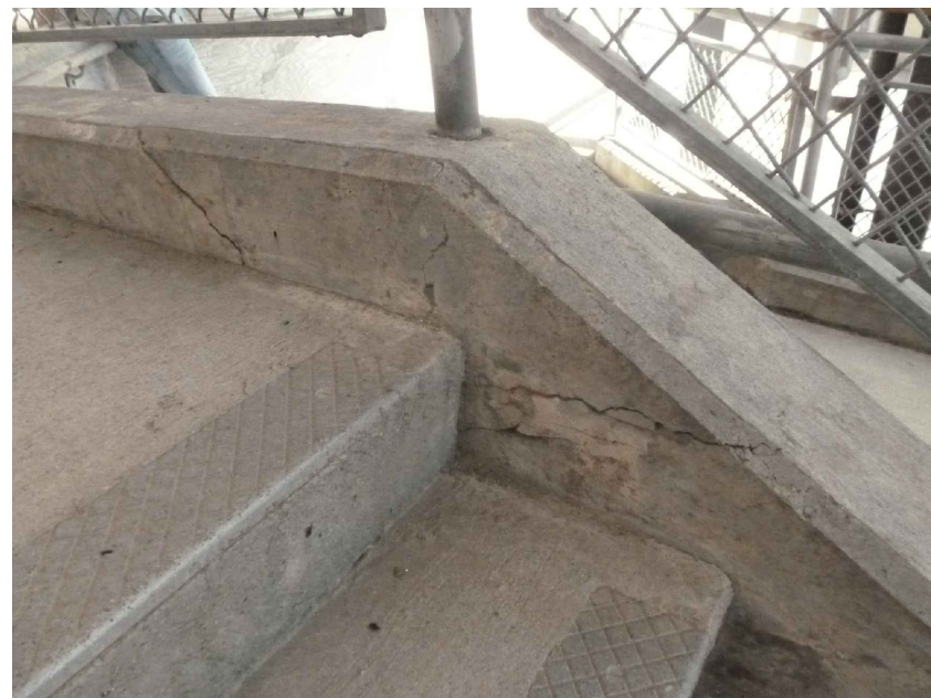
PH2 RAMP WALL CRACK
